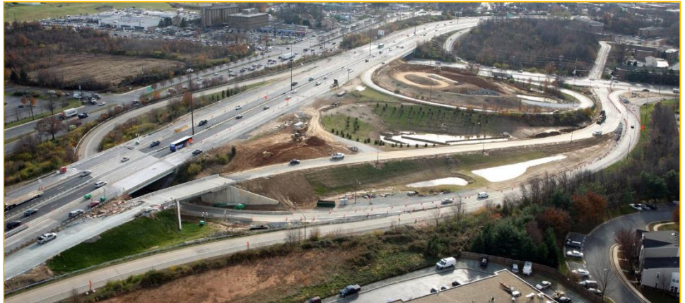
ICC-A facing west toward western terminus of ICC project over MD355-I-370 interchange including two bridges on the left
