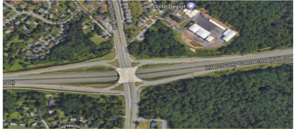
MD 650 SPUI Bridge
